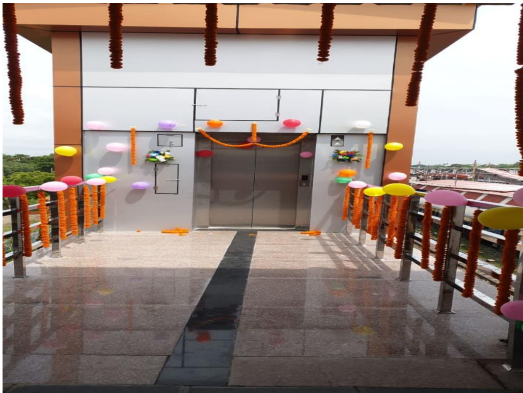
Lift at PF No. 6&7 at Gaya
