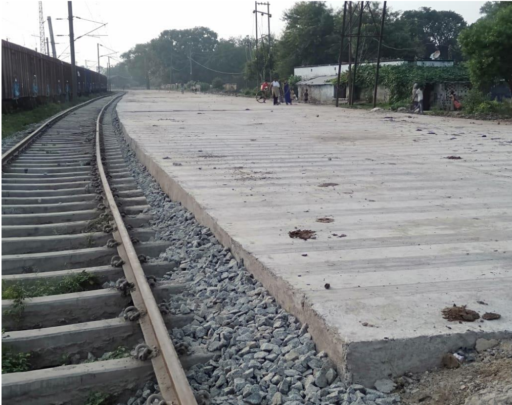
Goods shed at Gaya
