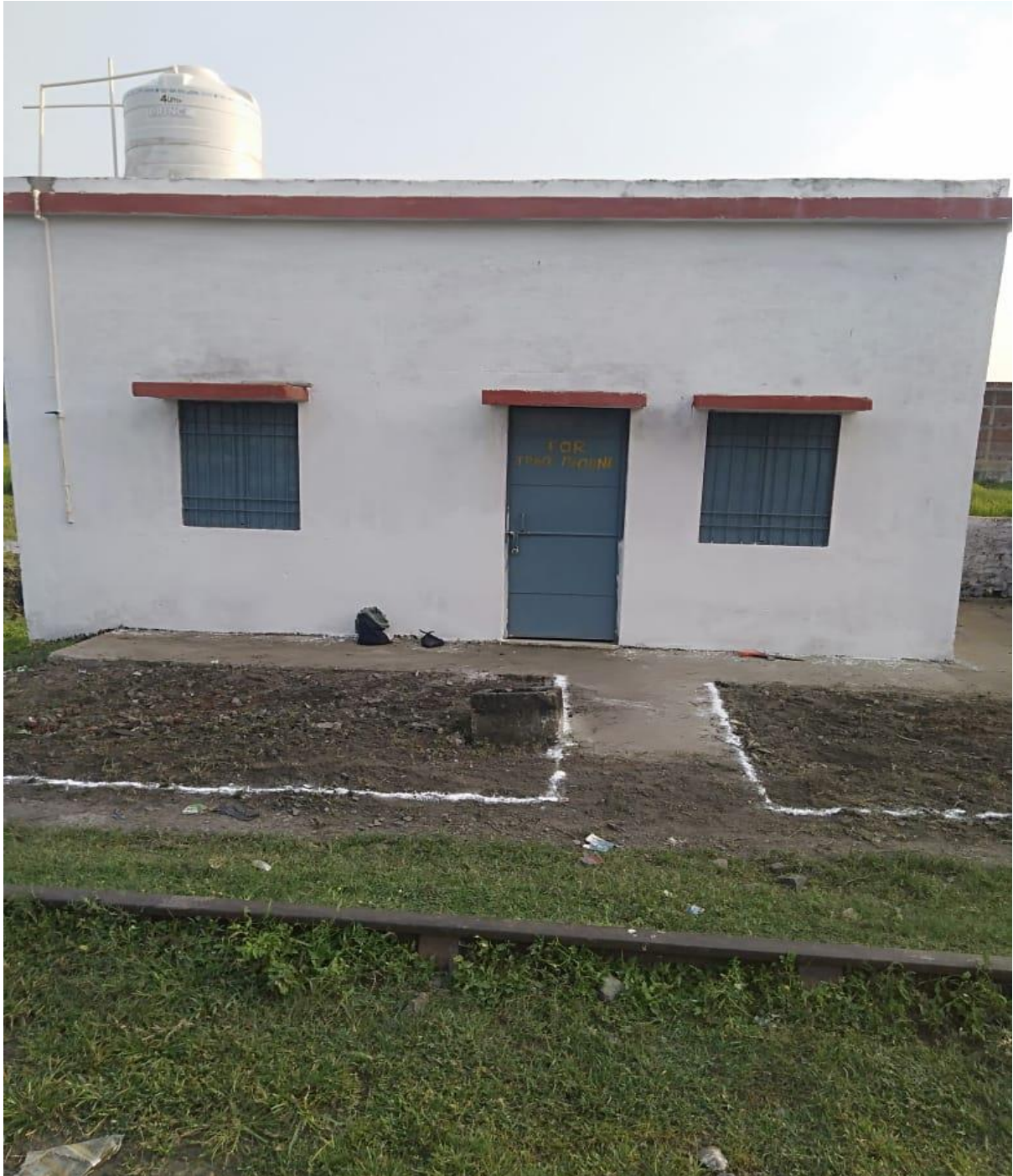
Rest room for Track machine siding at GRRU
