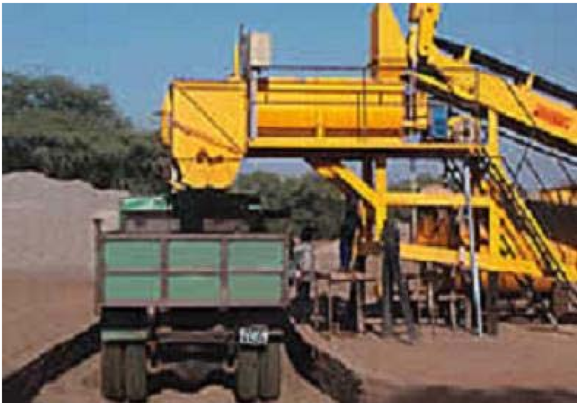
BLANKET MATERIAL BEING LOADED INTO TRUCK
