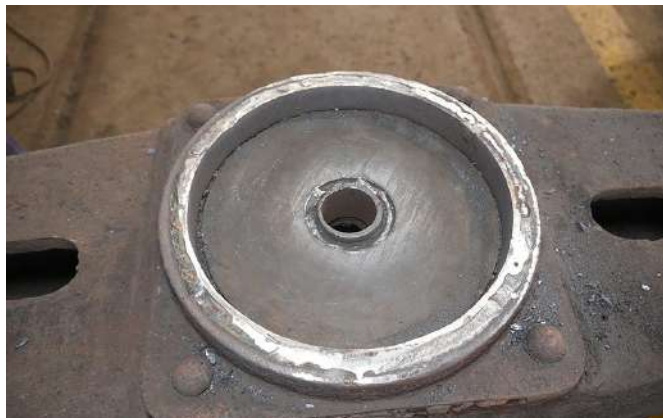
Figure16 Flat CP-after liner fitting & welding
