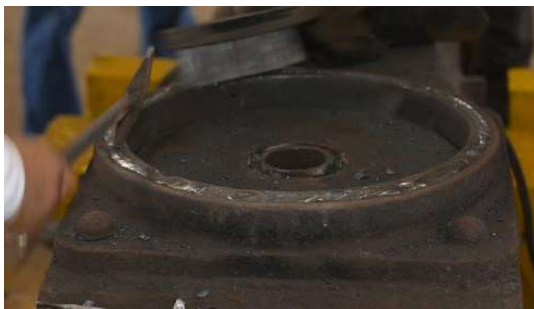
Figure 7 Flat CP- new liner welding
