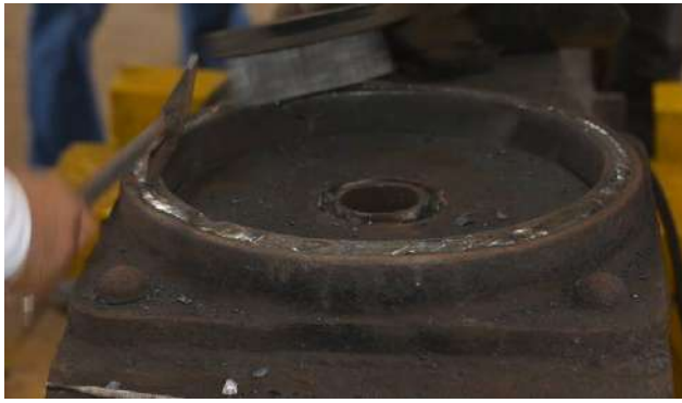
Figure 10 Flat CP- new liner welding
