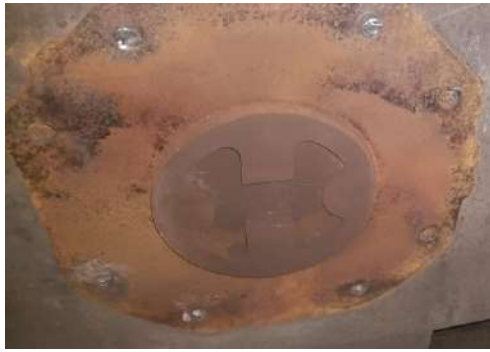
Figure 23 Flat CP top mounting location examination- Surface shall be examined for any crack etc. and attended as per relevant repair procedure of body bolster for respective wagon
