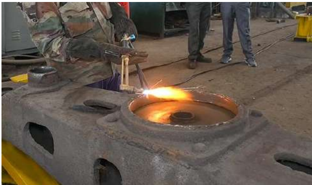
Figure 6 Flat CP liner removal(Damage to CP should be avoided)
