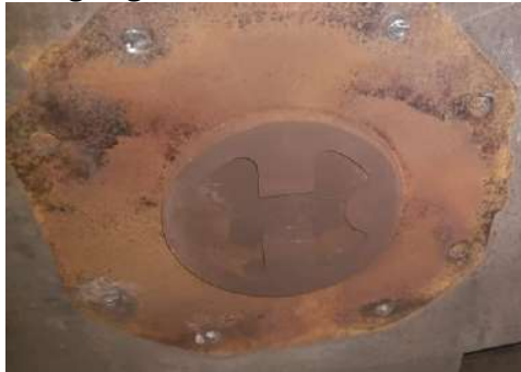
Figure 20 Flat CP top mounting location examination- Surface shall be examined for any crack etc. and attended as per relevant repair procedure of body bolster for respective wagon
