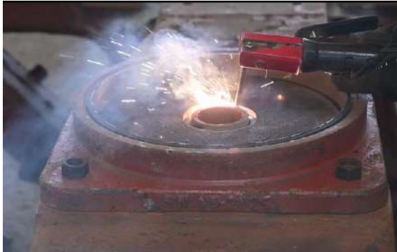
Figure12 Flat CP- horizontal liner complete welding all along the periphery as per the drawing. Post welding top surface of liner should be free from any burrs, weld projection etc. which shall be grinded
