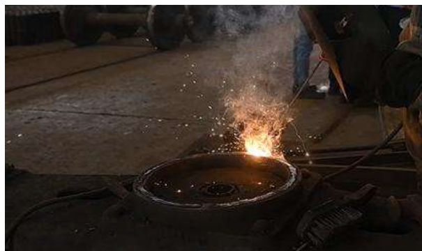
Figure 6 Flat CP- vertical liner complete welding all along the periphery as per drawing
