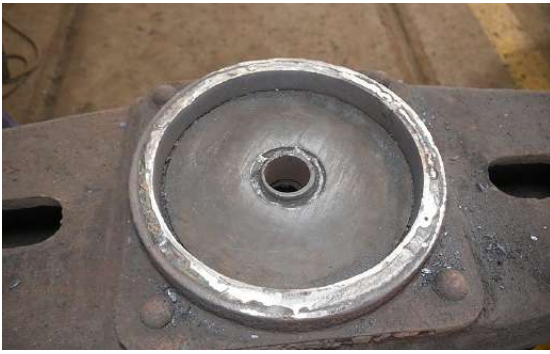
Figure 13 Flat CP- after liner fitting & welding
