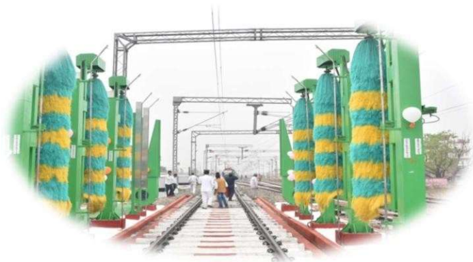
AUTOMATIC COACH WASHING PLANT
