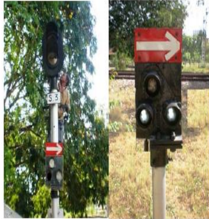
Shunt signal below stop signal Shunt signal on independent post
