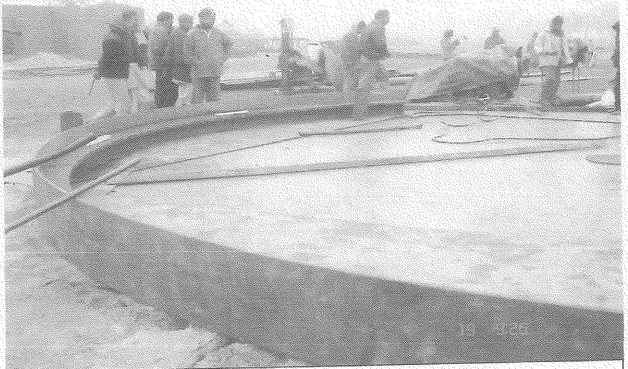
Fabrication of Cutting Edge of Well for A-2 in Progress
