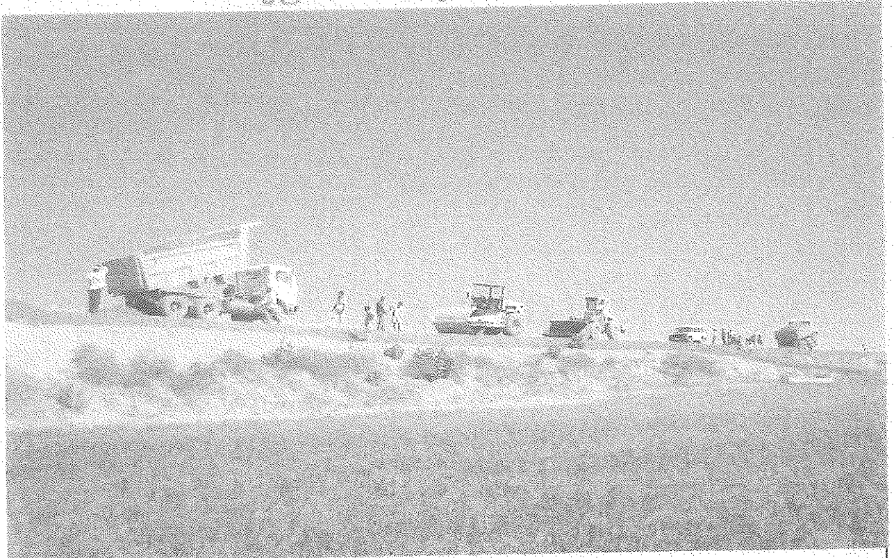
Blanketing Work in Progress
