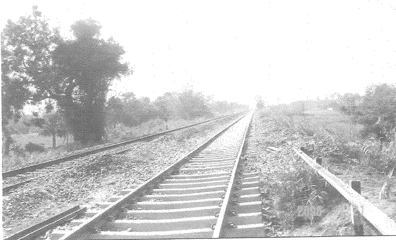
Track Linking In Progress
