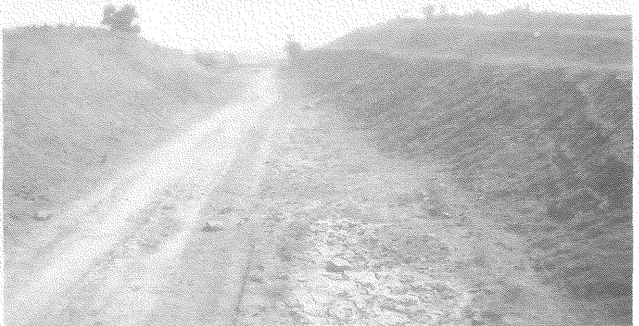
Earthwork in Progress
