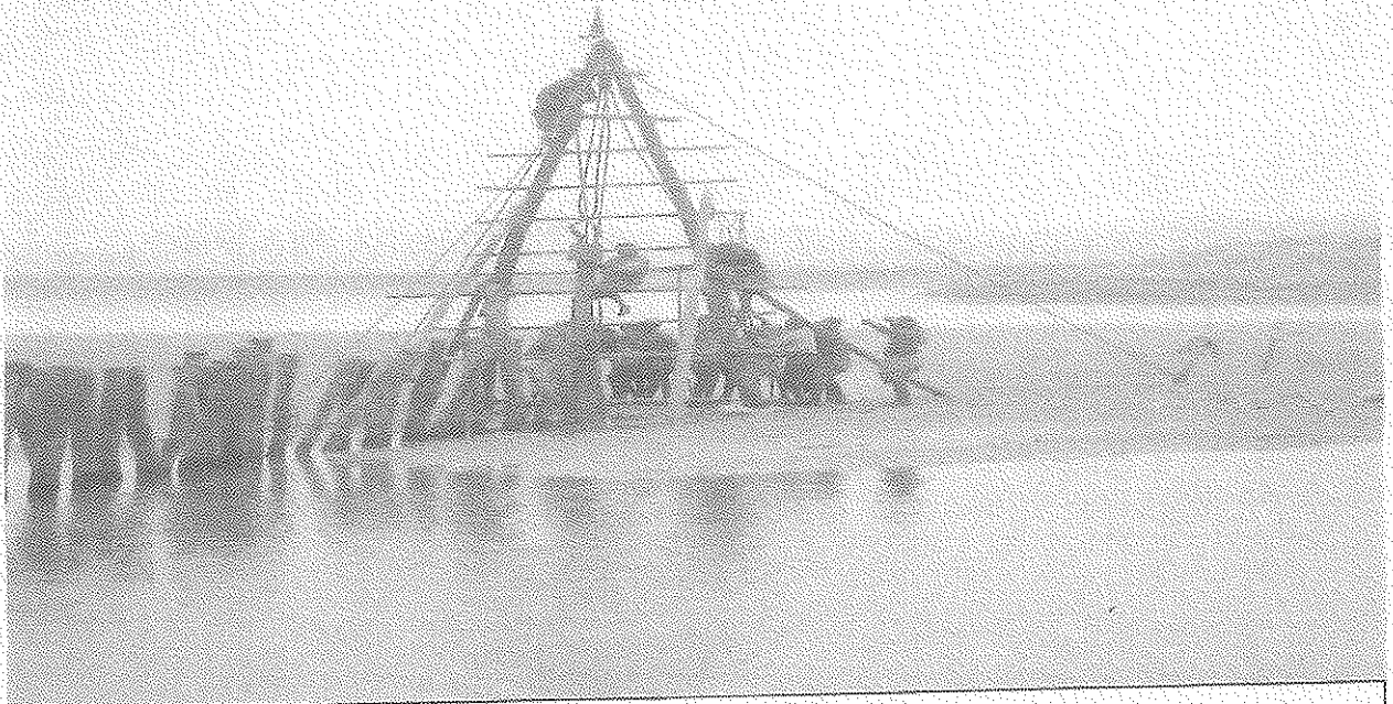
Blocking of River Channel for Construction of Approach Road in Progress
