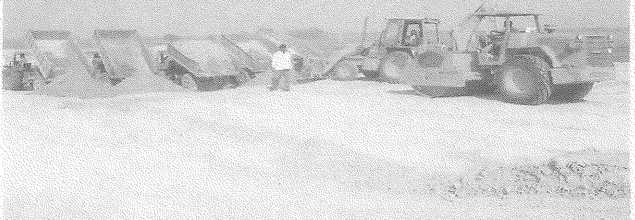
Earthwork In Progress
