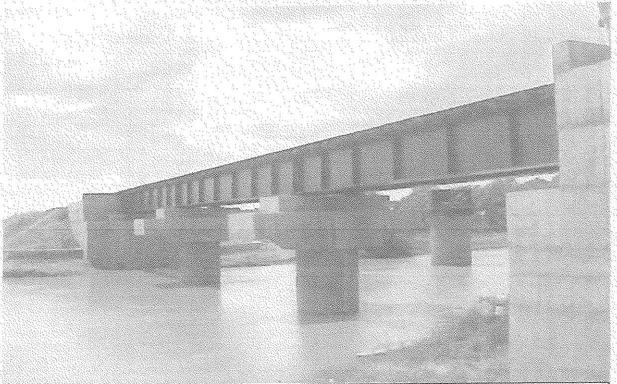
Construction of Major Bridge in Progress
