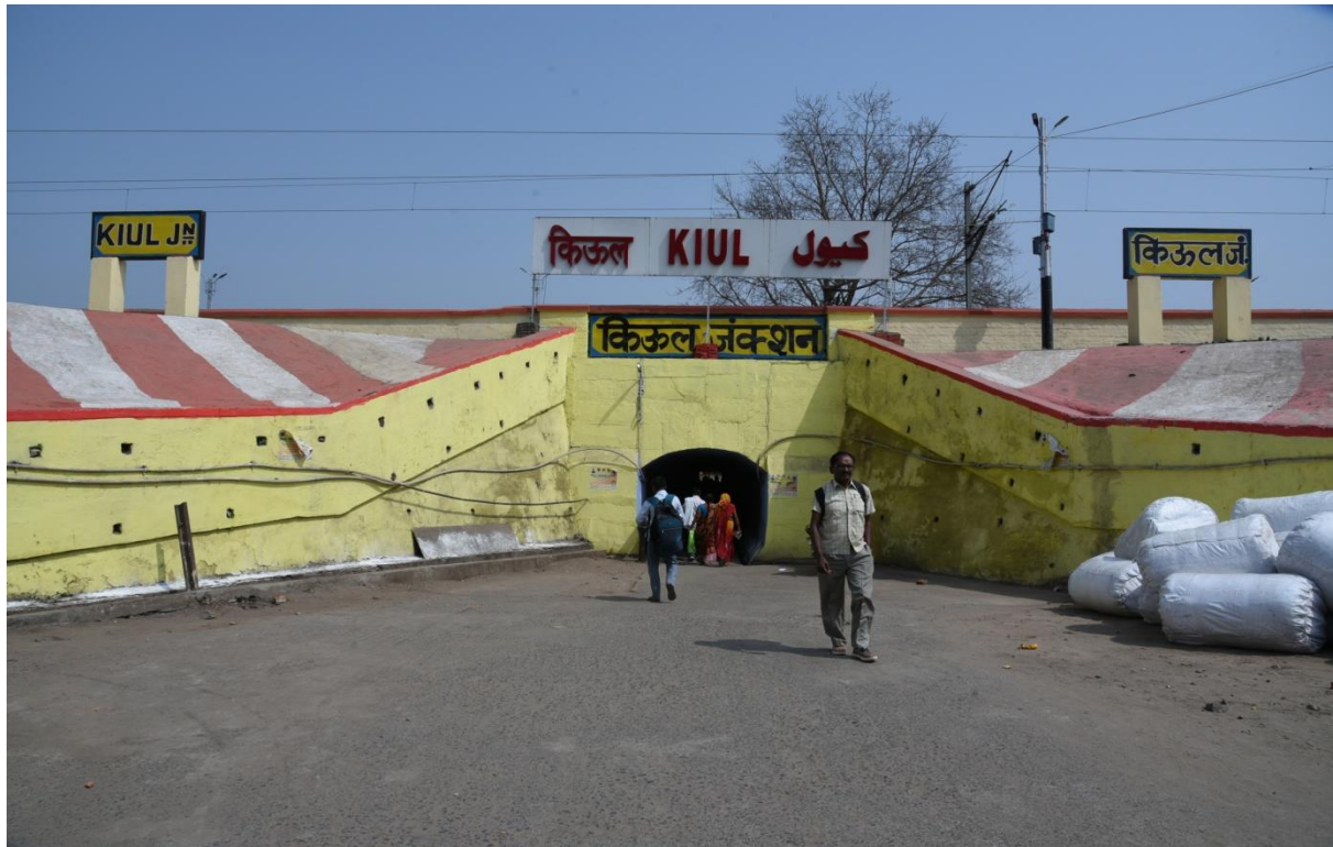
DNR 2 under pass connecting platfor at Kiul Station
