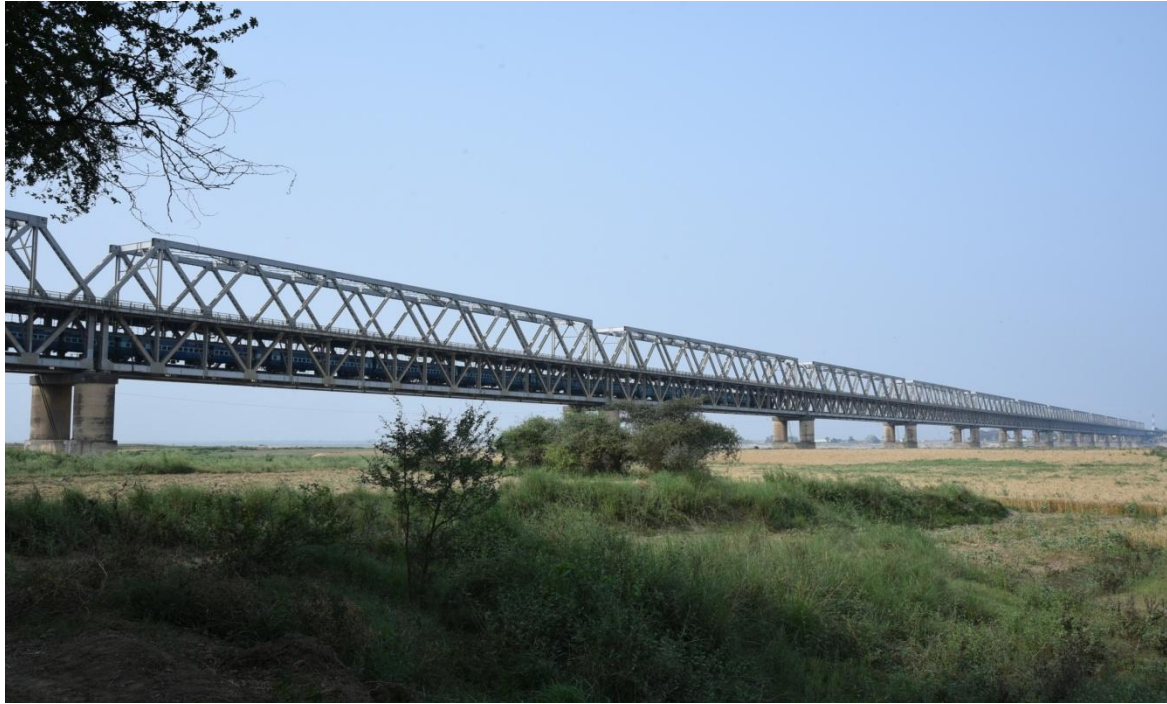
DNR 41 Rajendra bridge at MKA constructed in the year 1956
