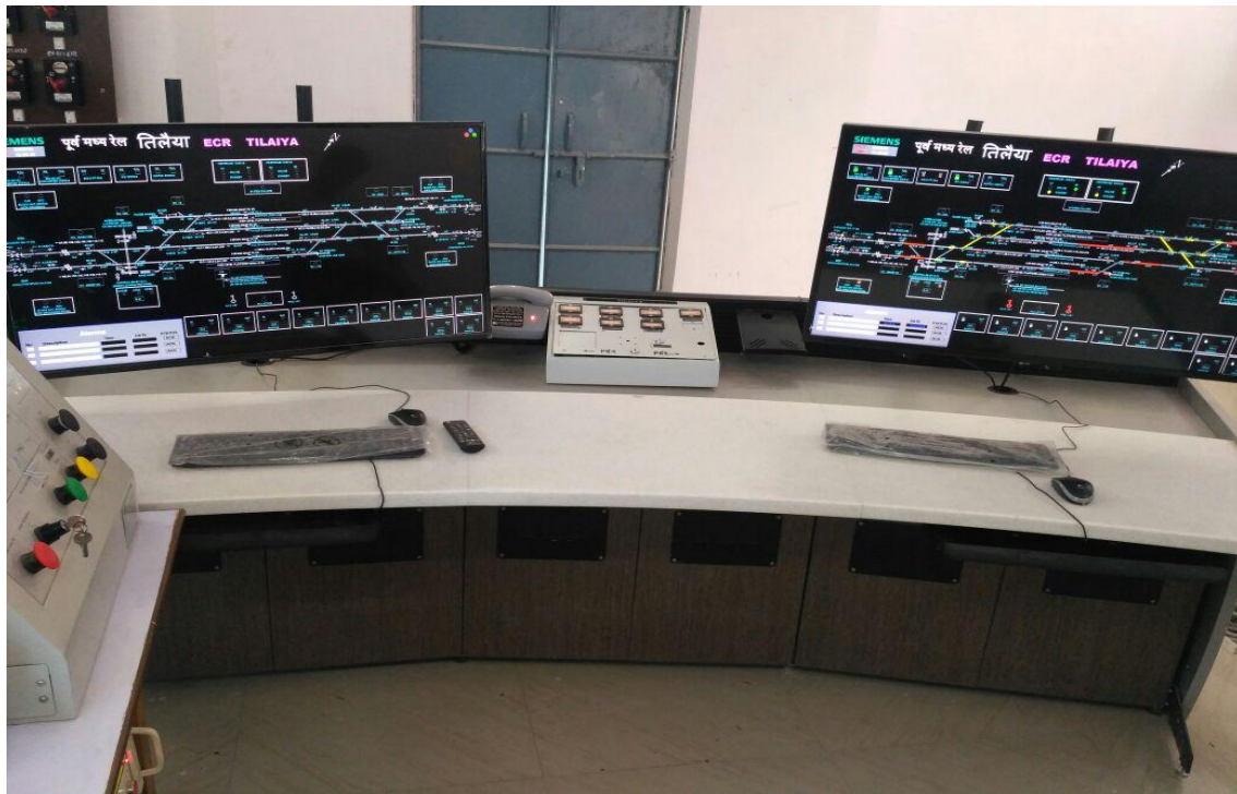
DNR 64 Electronic Interlocking Tilaiya
