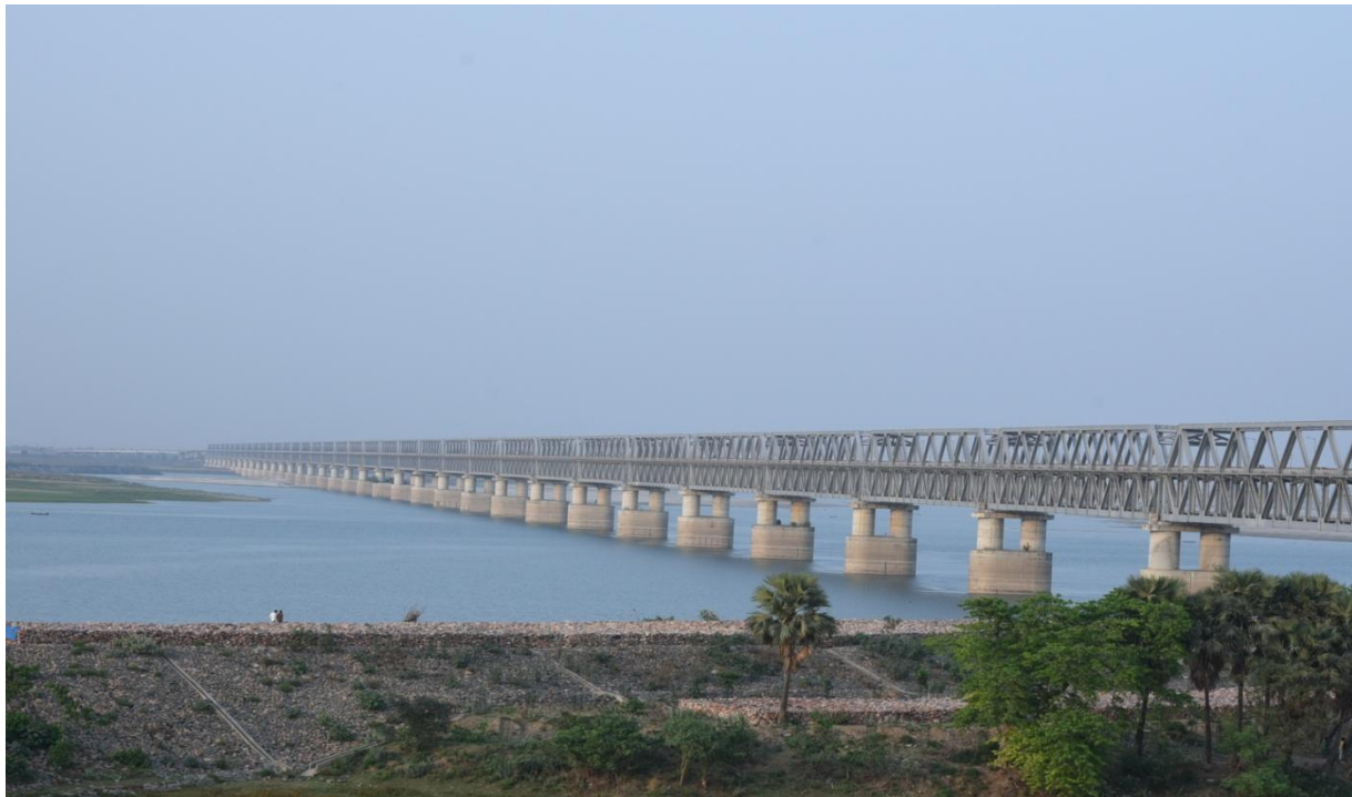
DNR 28 Digba Rail Cum Road bridge built in 2014
