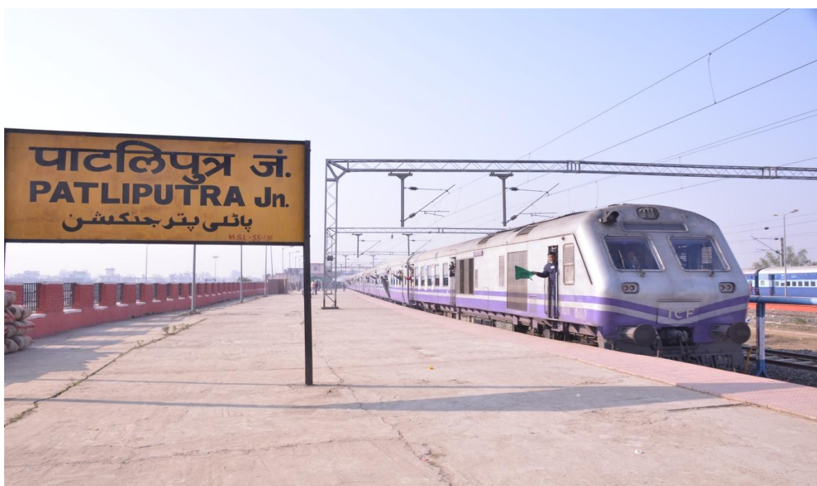
DNR 30 Operationalisation of Patliputra station
