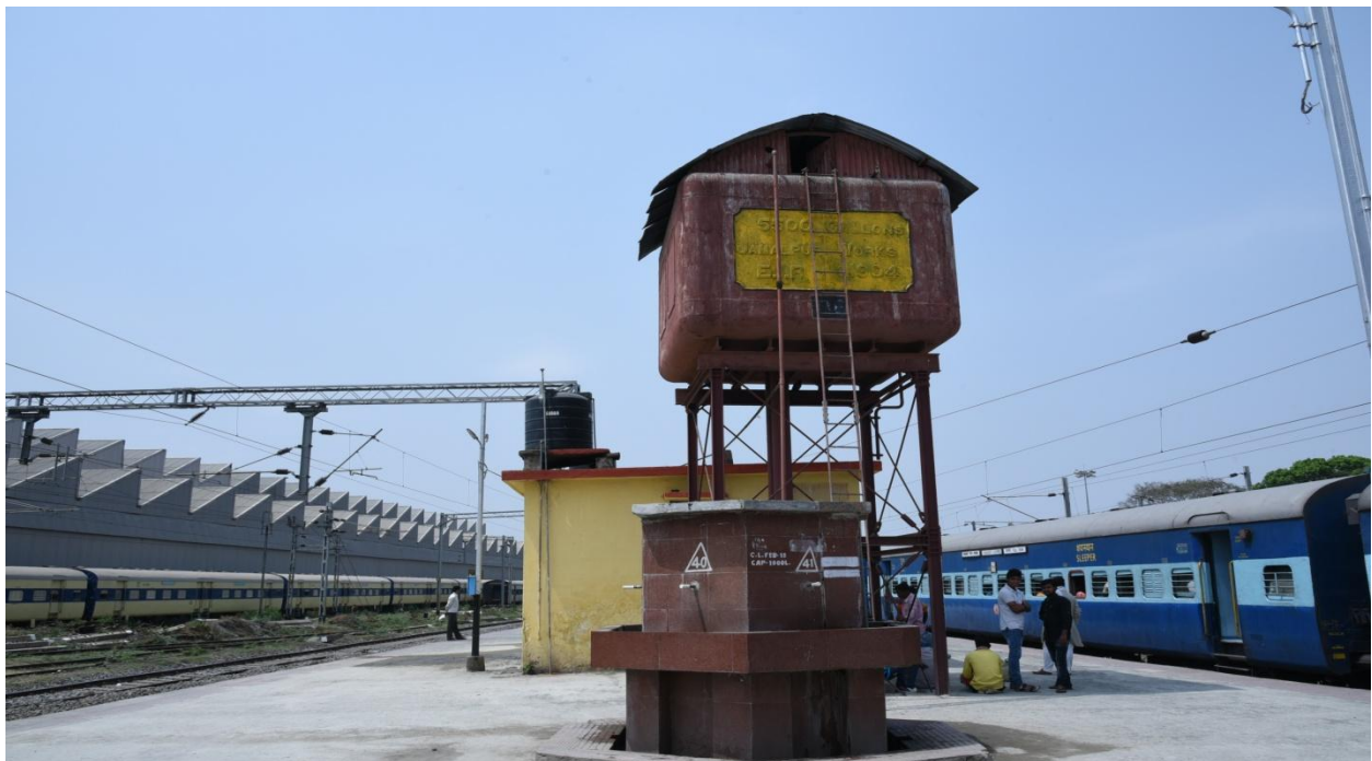
DNR 26 Jhajha station Water tank built 1904
