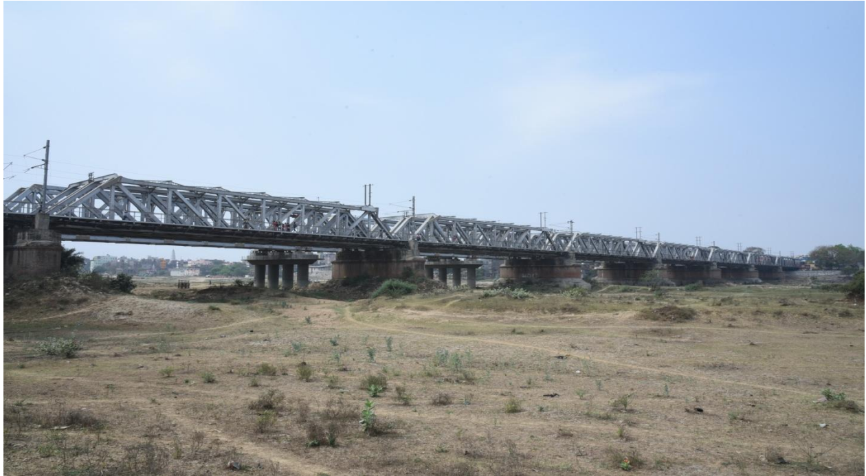
DNR 23 Kiul Rail Bridge constructed in the year 1910
