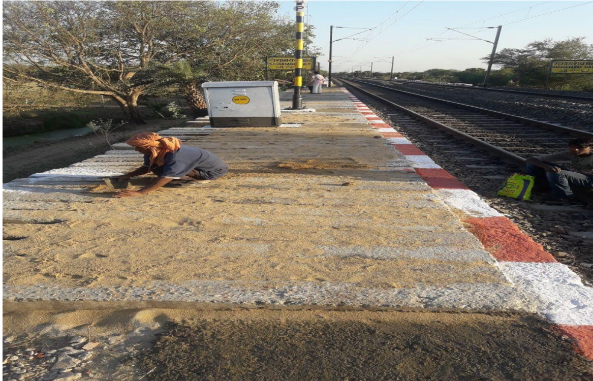
DNR 43 Construction of platform by release sleeper at Ganga Sarai Halt
