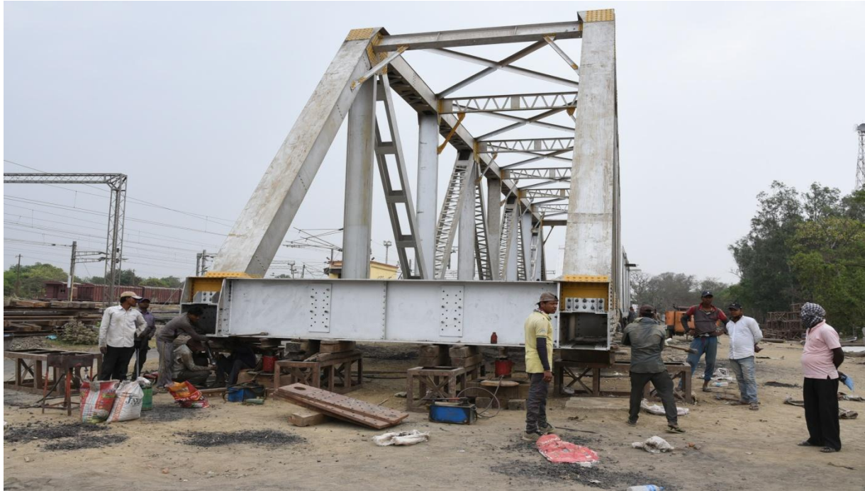
DNR 25 New Kiul bridge under construction
