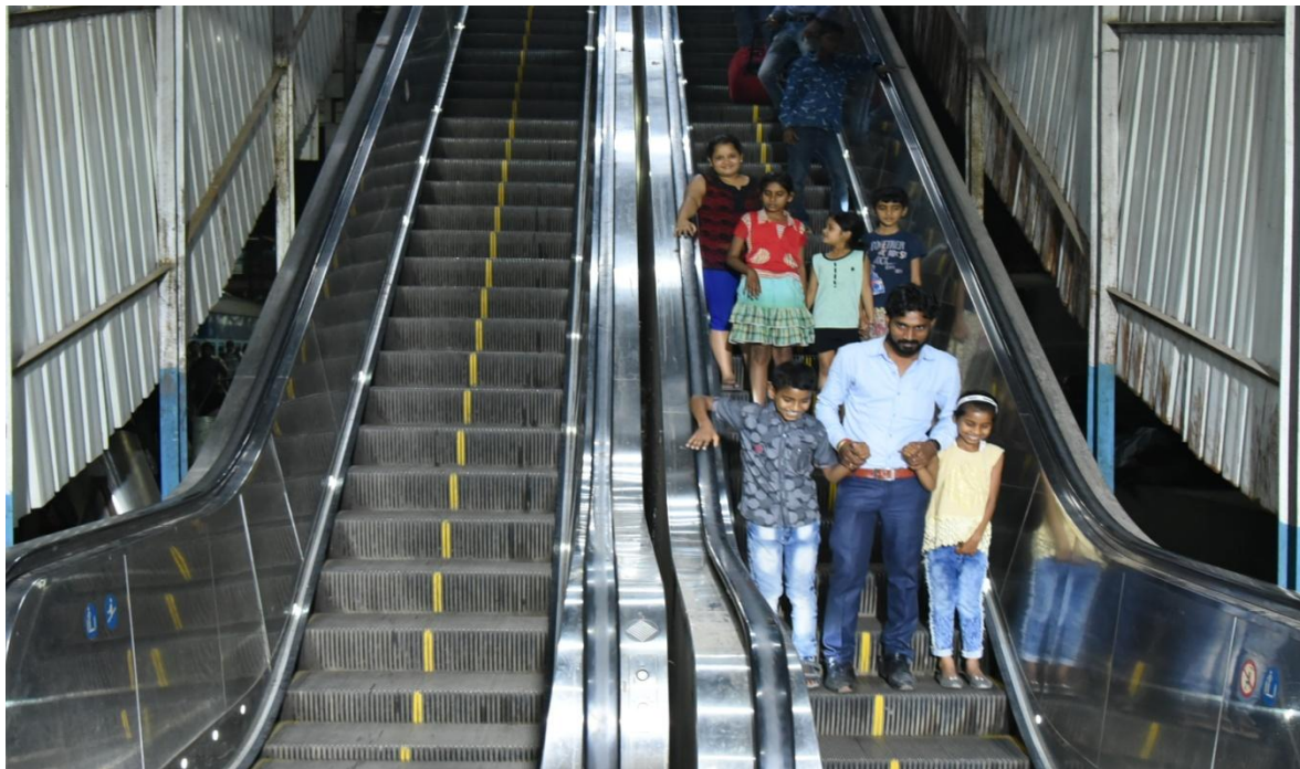
DNR 32 Escalator service provided at Patna
