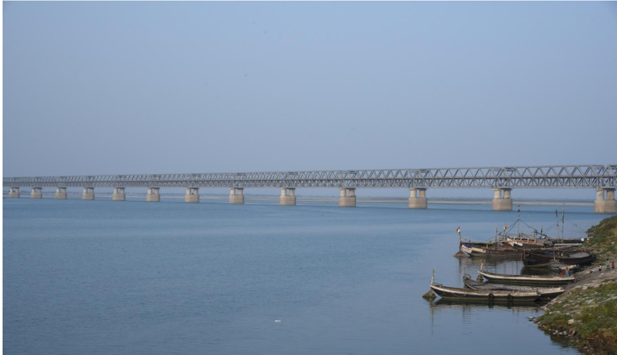
DNR 29 Digba Rail Cum Road bridge built in 2014
