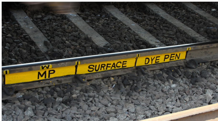
Fig. 28: A Typical Test Site on SCR
