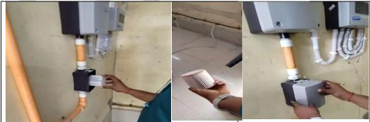
v. Detach the sampling pipes and use compressed air to clear out dust or debris. (This should be performed once every quarter.)
